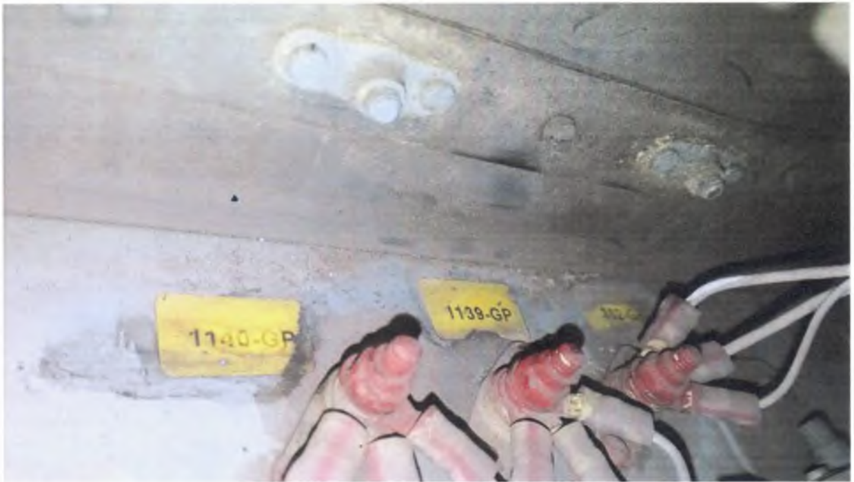
Figure 4. Ground point 1140-GP, 1139-GP, 382-GP.
